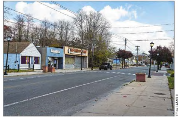
The Neighborhood Road business district is getting a face-lift.
